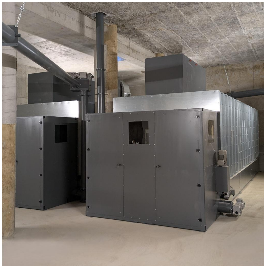
Example installation of two dryers in the negative pressure version with hoods.
